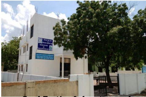
Seed Testing Laboratory and Training Complex at Raichur
